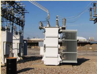
Three-Phase Transformer Single Unit, Substation Type
